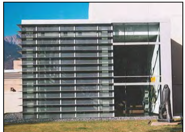
This building uses overhangs on the windows to provide shade in the summer months, but maximize solar access in the winter.
