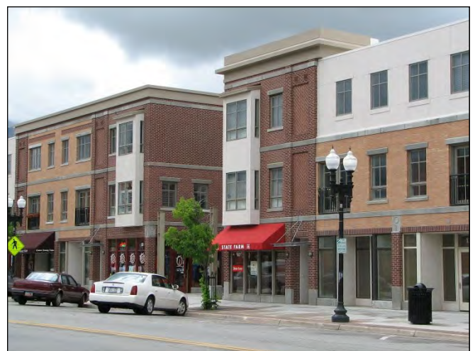
Synthetic stucco or exterior insulation and finishing systems (EIFS) are discouraged and do not qualify for this guideline.
